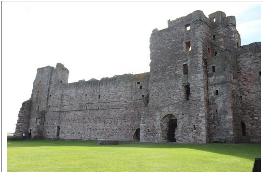
The interior of the landward wall at Tantallon Castle, featuring the east tower (left) and central tower (right). The two lines of square holes in the lower part of the wall show where ancillary buildings - possibly a stable block - would have stood when the castle was in use as a residence. Image source: Yours truly.
