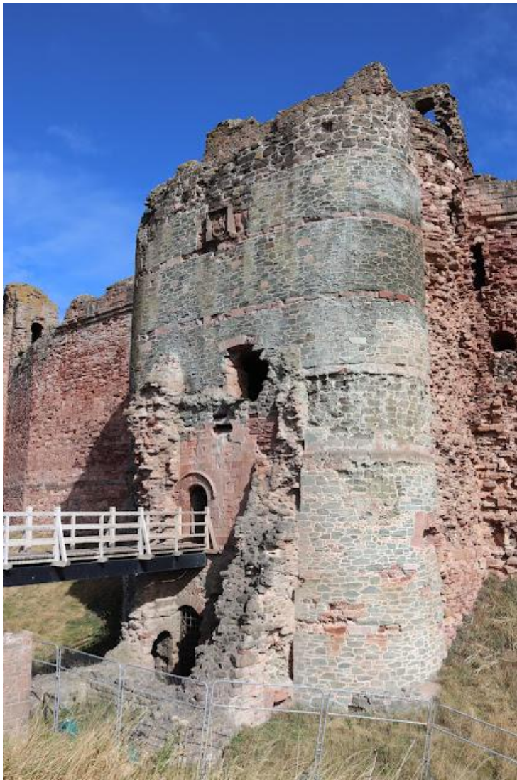
The barbican at Tantallon Castle. This part of the castle apparently bore the brunt of the damage during the siege of 1528, resulting in it being rebuilt and remodelled. The rebuilding work was undertaken with greenish basalt stone and can thus be seen quite clearly when compared to the areas of original red sandstone. The walls would have been harled - i.e., limewashed - when the castle was still in use, and so the different stonework would not have been so obvious. Image source: Yours truly.
