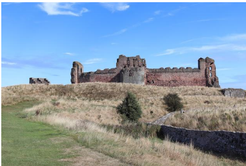
Earthworks at Tantallon Castle. The existing ditches and banks most likely date to the castle's final siege in 1651, but comparable earthworks were probably a major part of the castle's defences throughout its history. Not only did these make it more difficult for enemy troops to approach the walls, they also increased the distance from which enemy artillery could fire at the castle itself and reduced the areas of the castle that could be targeted by them, as this image demonstrates. Image source: Yours truly.
