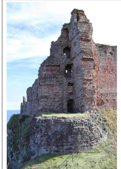
The west tower, known as the Douglas Tower because this was most likely the main residential block of the castle. Five of the seven storeys can be seen here, while the remaining two are located behind the remaining revetment in the lower part of this image. While they have been exposed to the elements since 1651, when the castle was in use these would have been some of the most sumptuous rooms in the castle, at times perhaps even in the whole kingdom. A partial inventory of the castle's furnishings from 1581 is a testament to this fact. Image source: Yours truly.
