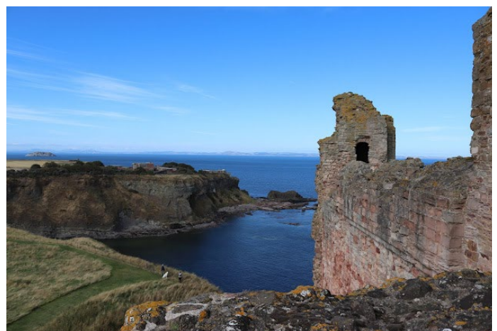
Looking east along the landward wall of Tantallon Castle from the forework of the central tower. Even a cursory appraisal of the defences at Tantallon vividly illustrates the futility of trying to assault the castle if a negotiated solution was possible, which no doubt explains Fife's actions in 1389. Image source: Yours truly.
